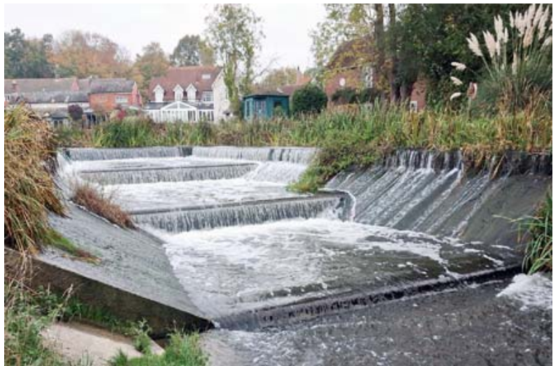
↑ It was pleasing to see the Horseshoe weir flowing once again in this photo taken on 12th October by Antony Day. The reeds will die down for winter as still no management of them has been carried out by the EA. The pipe that was inserted to help with a little flow over summer was still there
