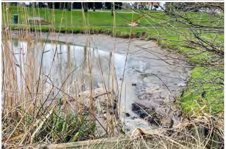
The pressure of water flow from the culvert has redirected the water flow around the reed bed and carved out a channel through the silt. The black layer beneath the lighter coloured silt is vegetation that has broken down; this clogs up the river bed.
