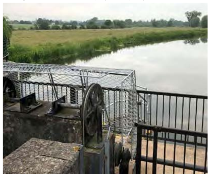
Photograph taken from above the sluice gates by Sally Dalton. The gates open to release water into the flood relief channel when river levels are high to prevent risk of flooding along the stretch of river that runs through the village.
