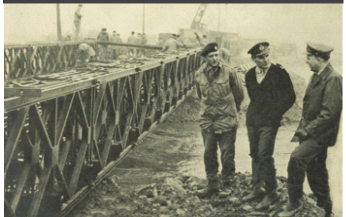
Royal Engineers erecting the Bailey bridge across the Stour, and below testing it with their lorries.
